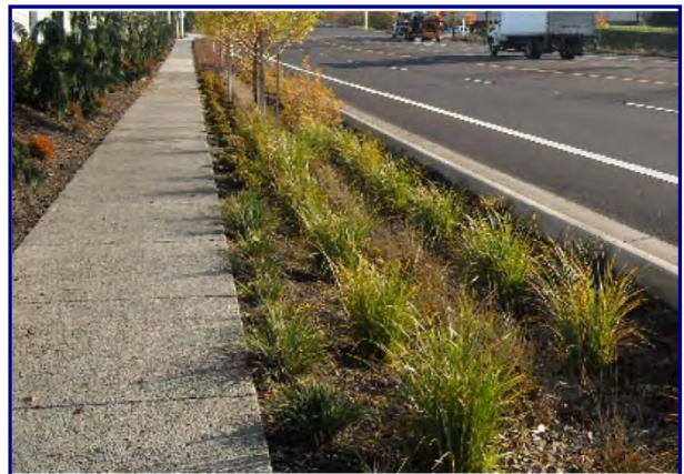
Example of Vegetated Swale along Street
