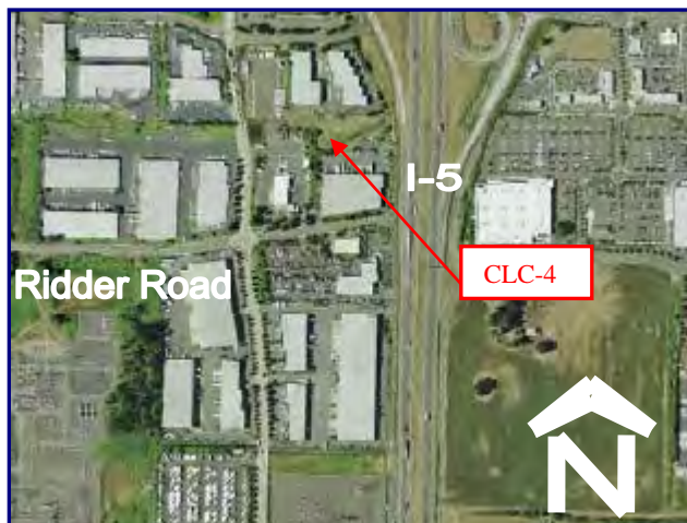
Aerial view of Project CLC-4
