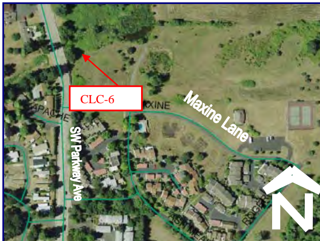
Aerial view of Project CLC-6
