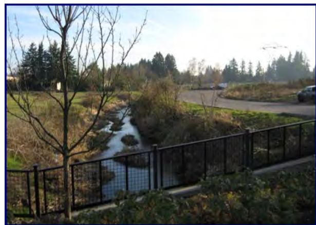
Looking south along Seely Ditch from Wilsonville Road
