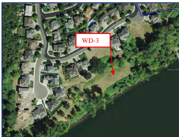
Aerial view of Project WD-3
