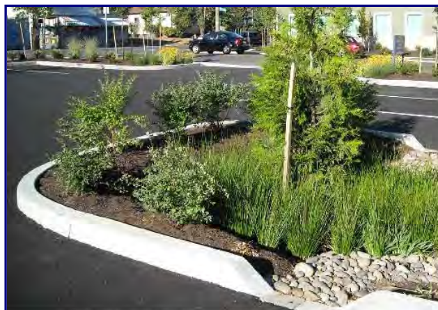
Example of Stormwater Planters in Parking Lot
