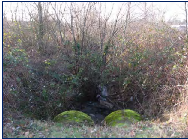
Looking West at Project SD4021 & SD4022
