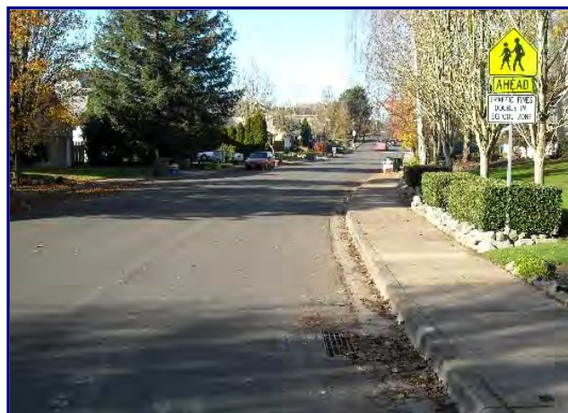
Existing Street Conditions
