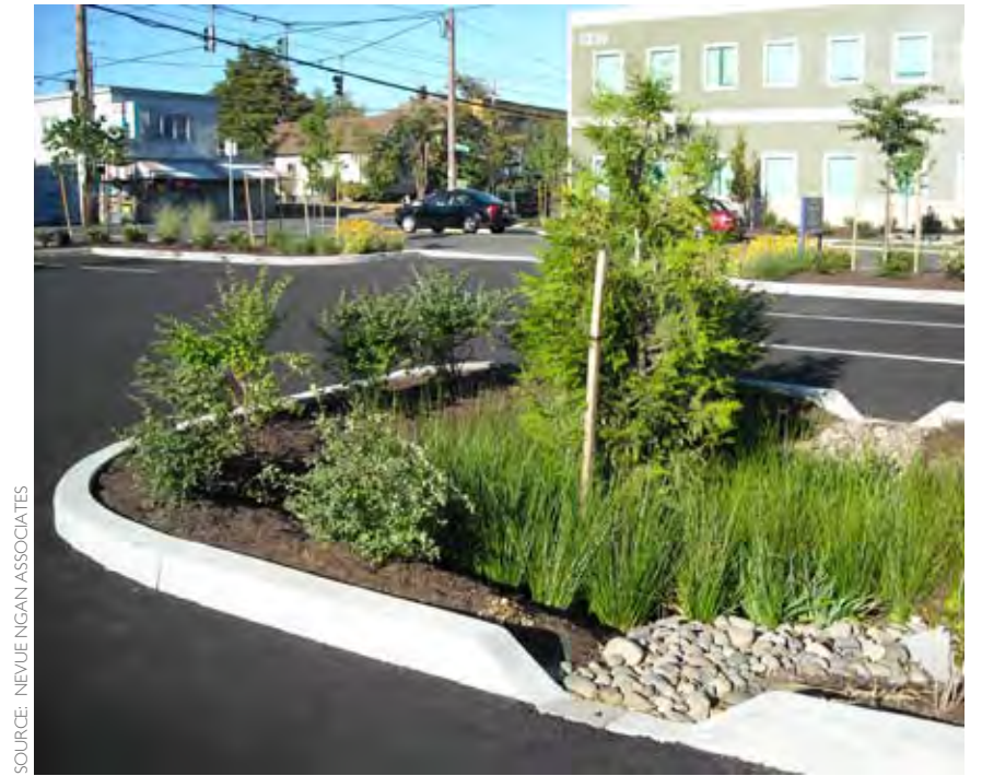
Example: Stormwater Planters
