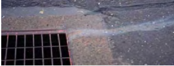
Figure #: When it rains pollutants are washed directly into pipes and then rivers and bays
