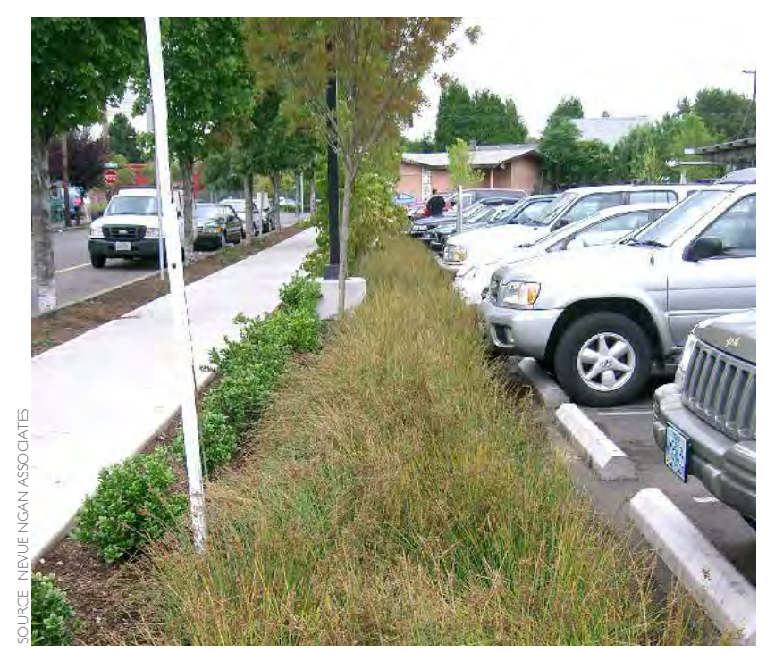
Example: A Green Gutter Within A Parking Lot
