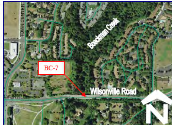
Aerial view of project location
