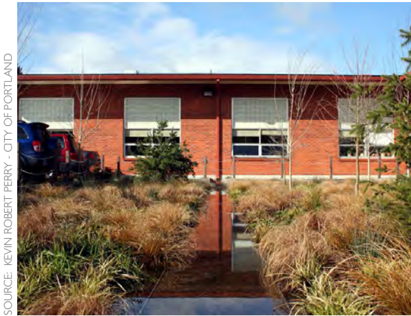
Figure #: Stormwater facilities filter sediments and other pollutants in runoff; which results in improved water quality.
