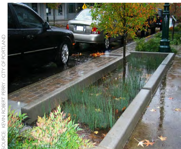
Figure #: Stormwater facilities collect and absorb stormwater to reduce the overall volume of runoff.
