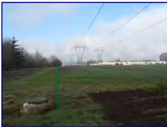
Looking west at the potential site of a stormwater detention pond
