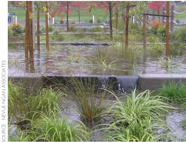
Figure #: Stormwater facilities slow the flow of stormwater runoff through the interaction of the water with plants and soil.
