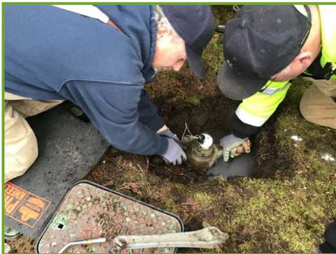
Water Technician's Chris Reece and Steve Gering replace the meter.
