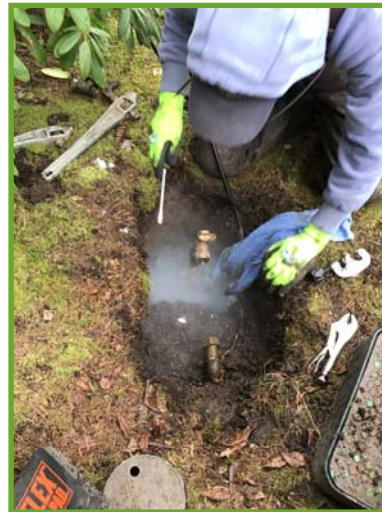
Water Technician Sam Kinnaman installs the new curb stop.
