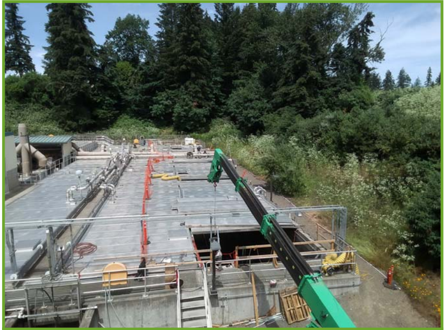
Crane removing cover panels over aeration basins
