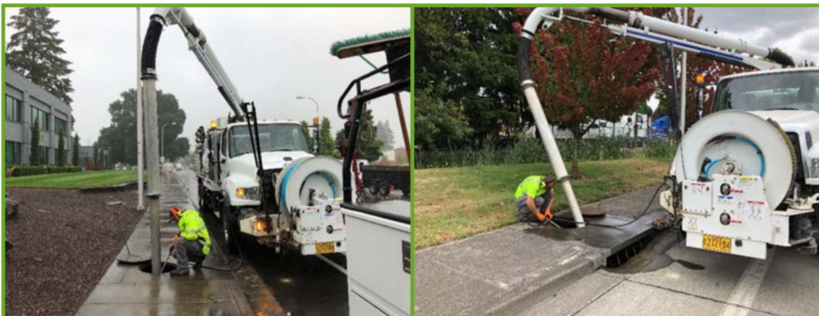
Performing scheduled catch basin cleaning
