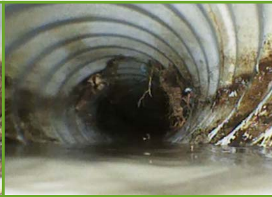
After— line cleared
