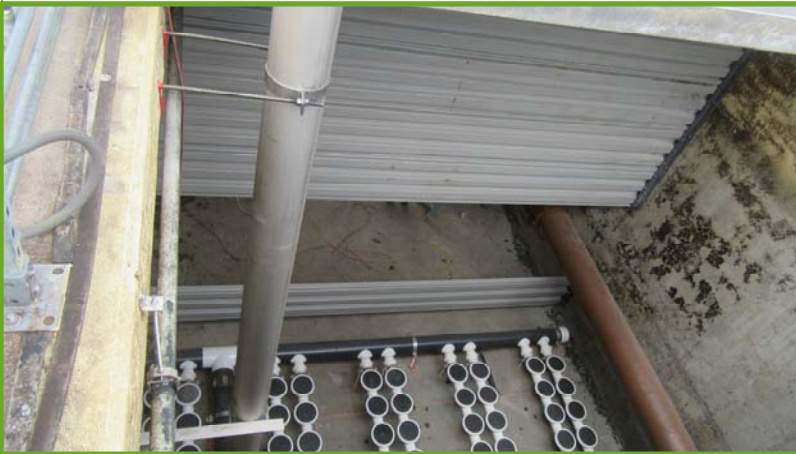
Relocated baffle wall to expand basin aerobic zone
