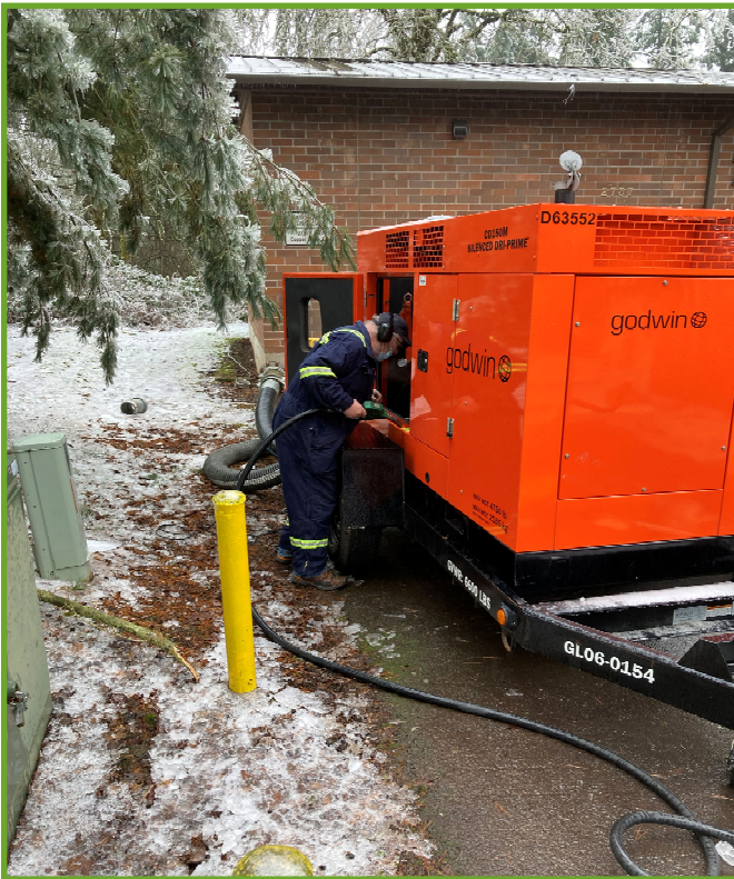
Refueling the portable pump
