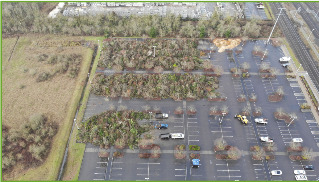
Before—Full debris drop off site looking to the north
