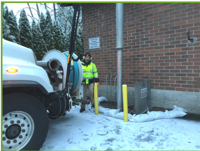
Jay Herber assisting at the lift station
