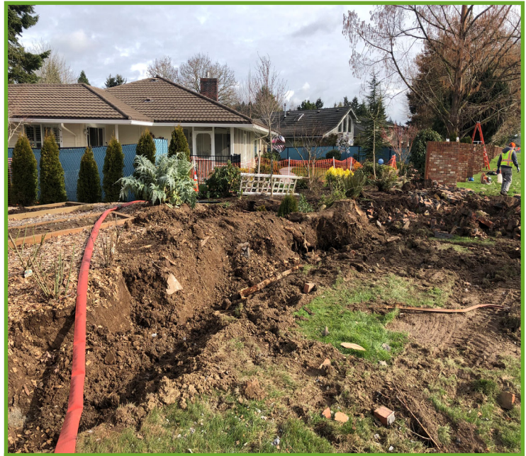
Miley Road Pipe Repair Project
