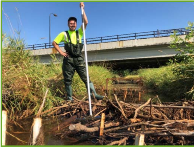
BEFORE— built up debris pile
