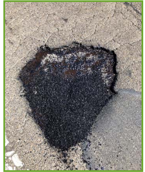
Newly filled pothole
