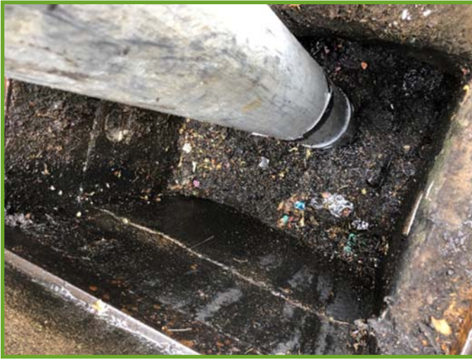
Before—no pipe in sight
