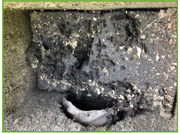
During—can start to see pipe
