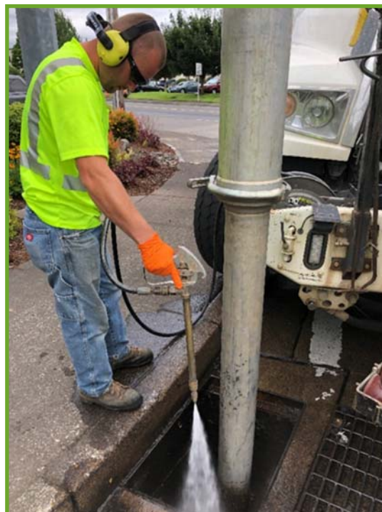
Cleaning catch basin
