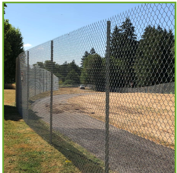
Construction fencing around the work area
