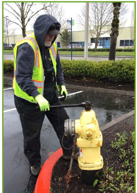
Steve Gering inspecting a hydrant
