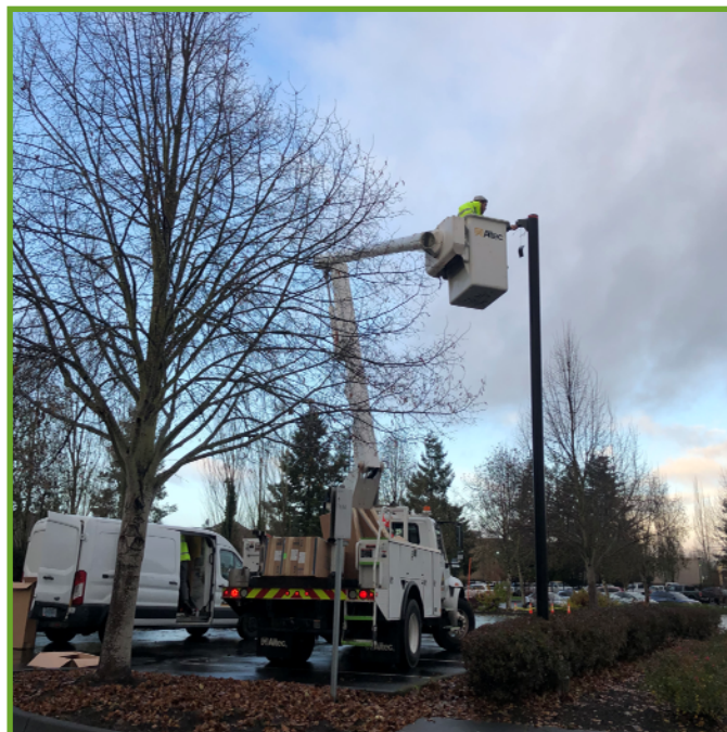
Upgrading light fixtures
