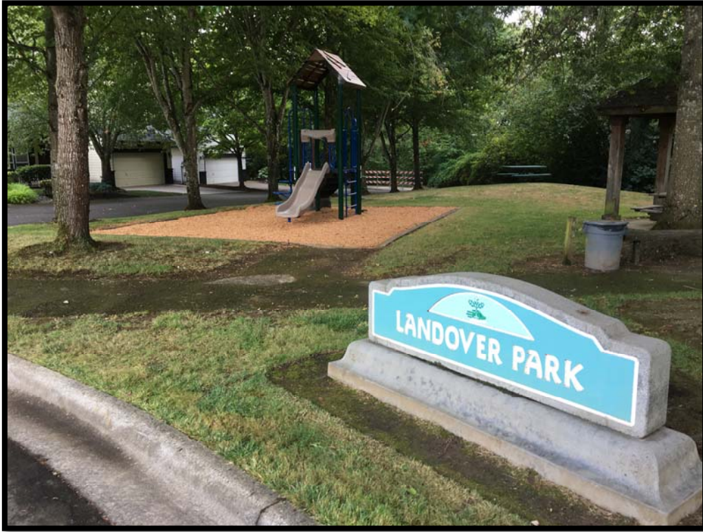
New Playground installation at Landover Park
