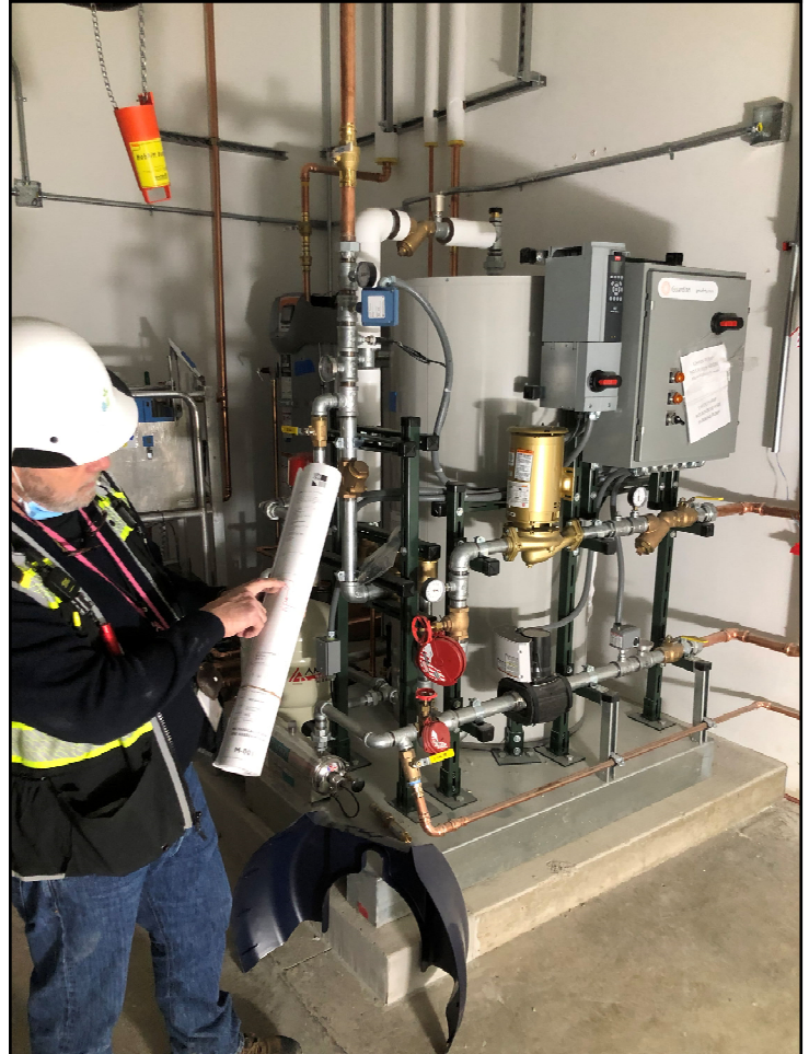
Building Inspector Mike Ditty on site at Twist Bioscience
