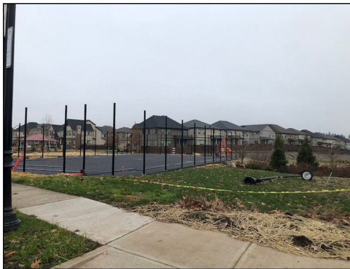
Tennis court fence installation.
