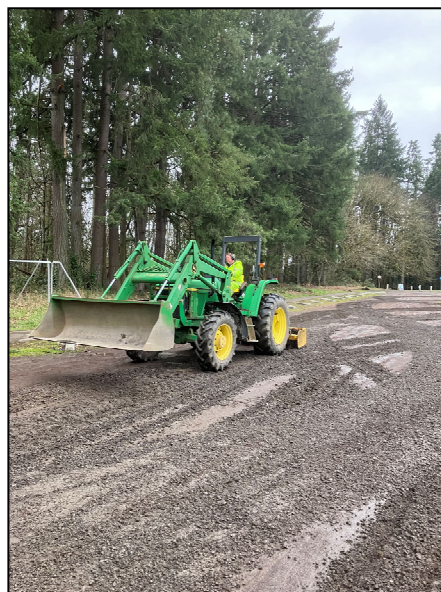
Parking lot grading.
