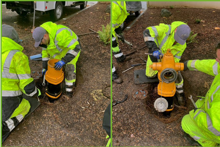
Replacing the damaged hydrant
