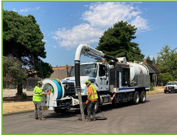
Jay & Tim cleaning a Stormwater manhole
