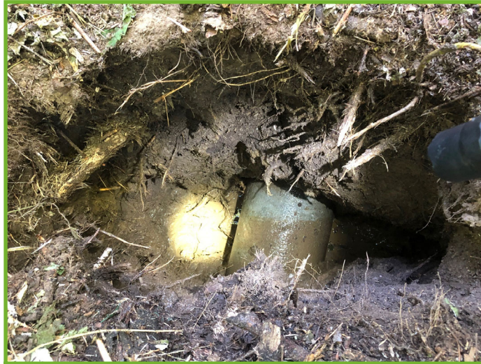
Potholing to expose pipe
