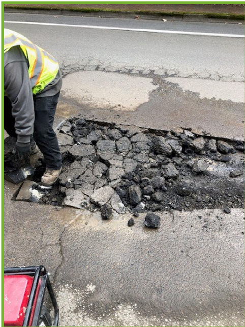
Removing the old asphalt
