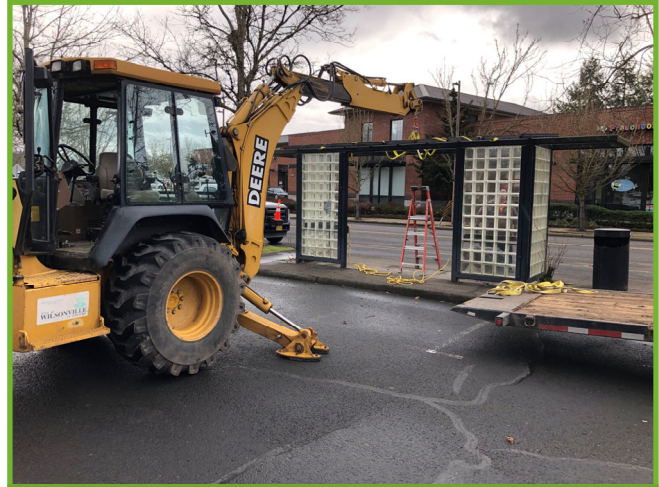
Securing to the backhoe
