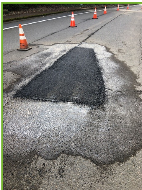
Patched and ready to be driven on
