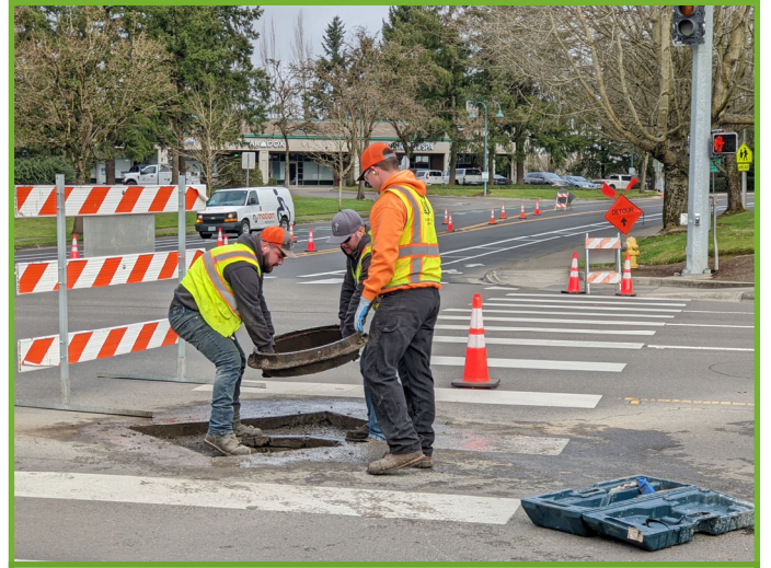
Setting the new metal ring in place
