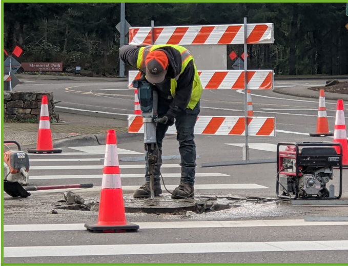
Removing the manhole and concrete collar
