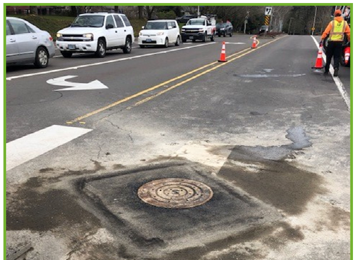
Finished project ready for traffic
