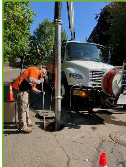
Cleaning water quality manhole
