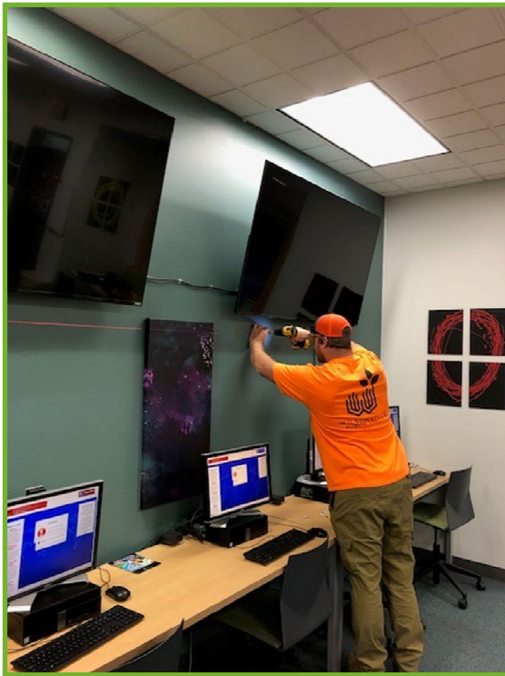
Installation in progress
