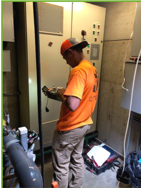
Konnen completes repairs
