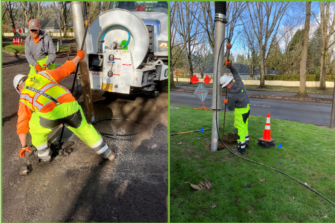
Performing 'potholing' to check water main size
