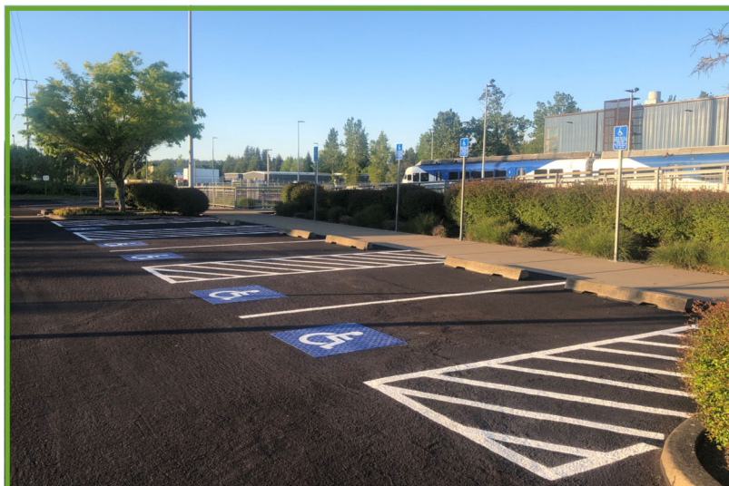
Fresh striping and surface at WES
