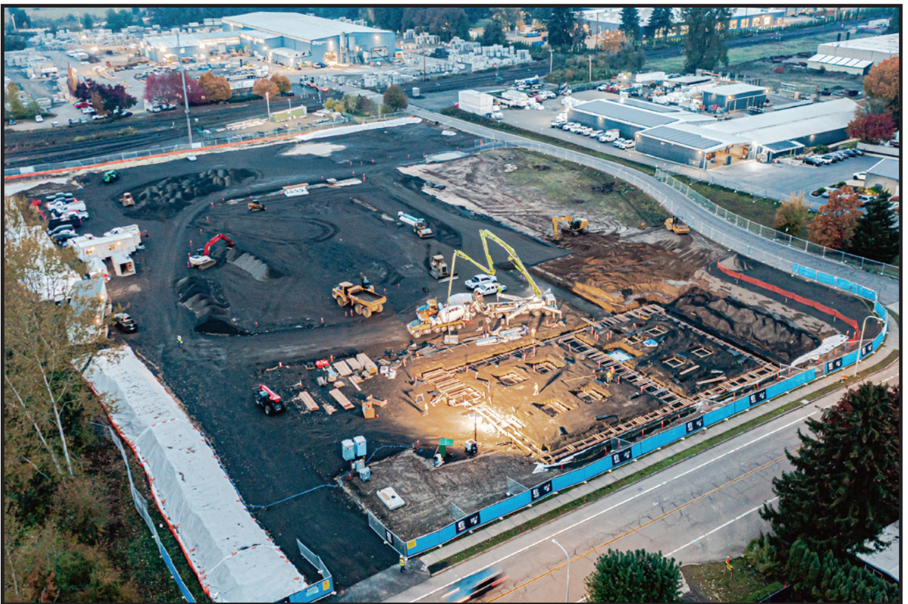
Construction begins on new Public Works complex. Photo credit: Emerick Construction.
