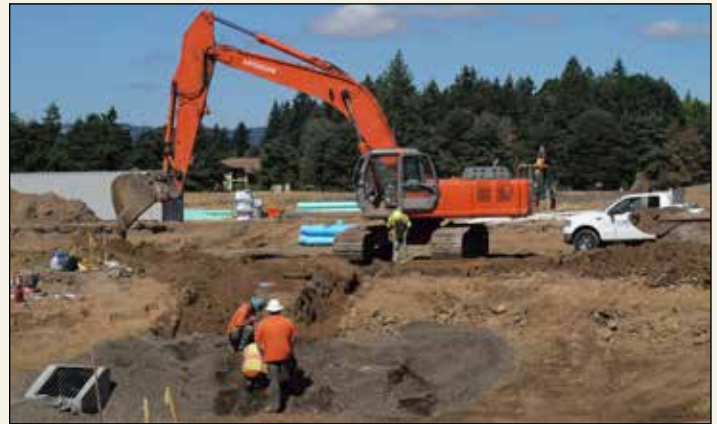
Contractors working on extending Canyon Creek Road.
