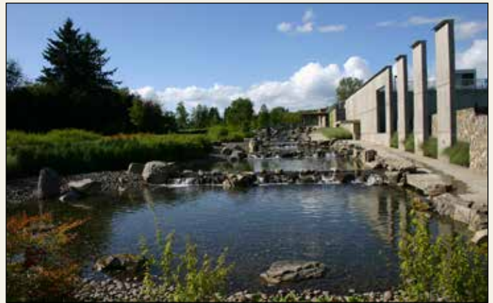
Water feature at the Willamette River Water Treatment Plant.
