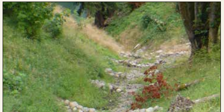
View of the Morey's Landing Stormwater Outfall project.
