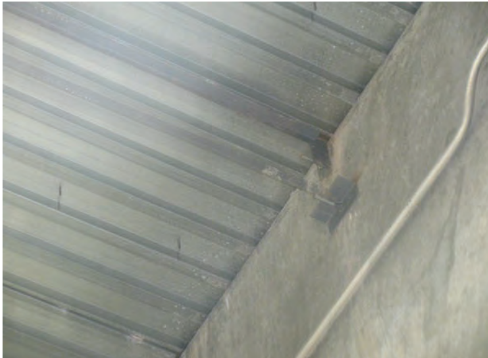
Photo 30 – S6 – Interior walls lack diaphragm shear capacity transfer from the roof diaphragm to the shear walls.
