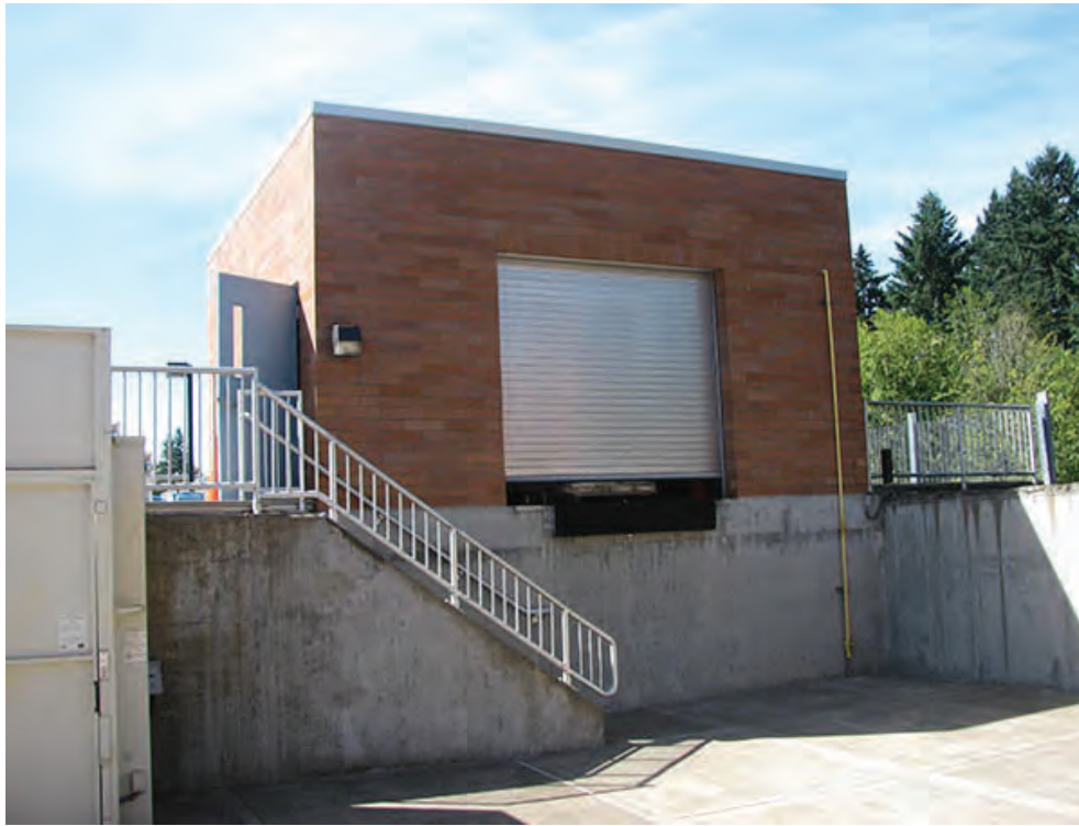
Photo 5 – LS3 – Guardrail at the north Actiflo™ staircase is less than 42 inches in height.
