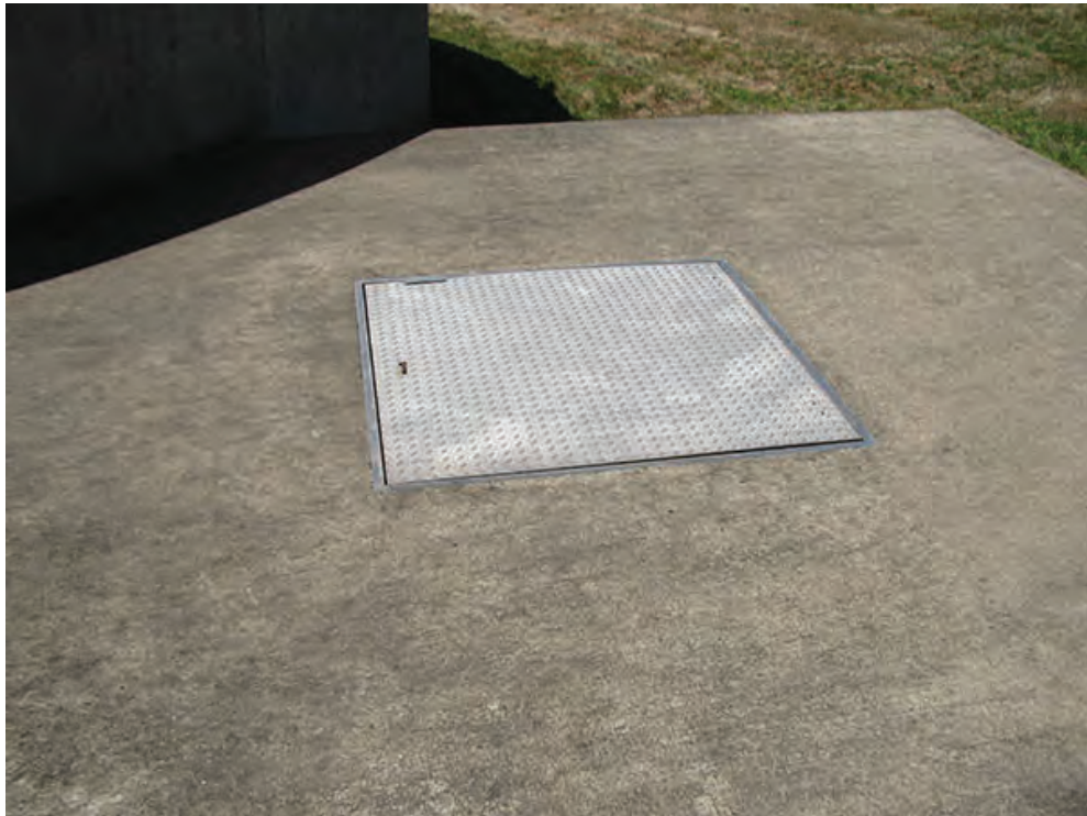
Photo 2 – LS1 – Access hatch at the Sludge Thickening PS as seen from the top side.
