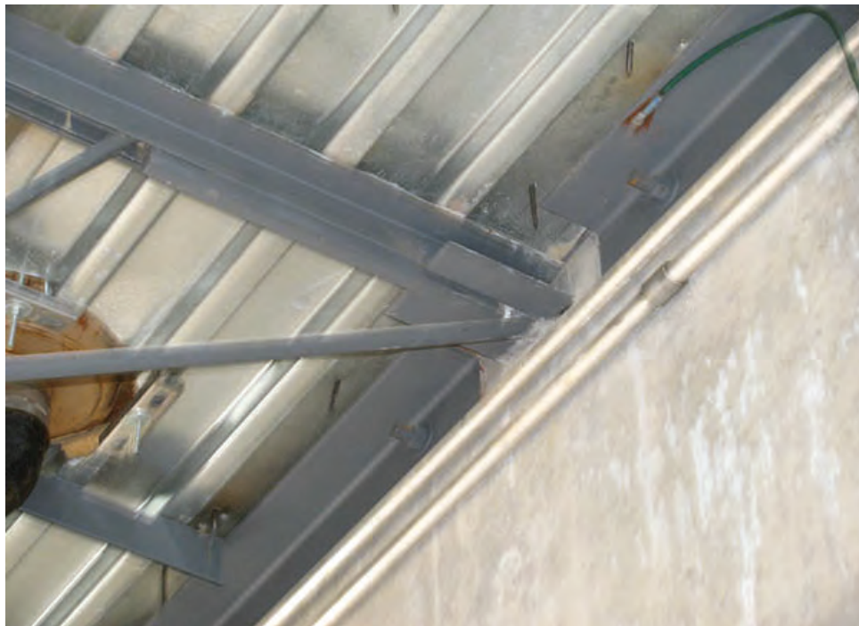
Photo 32 – S8 - The roof joist wall anchorage to the walls at the Solids Dewatering Building lack capacity to meet seismic performance goals.
