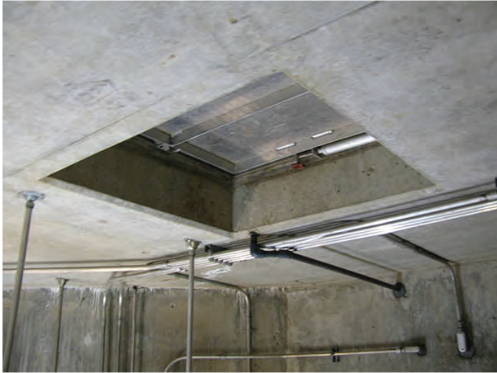
Photo 1 – LS1 – Access hatch at the Sludge Thickening PS as seen from the underside of the concrete deck
