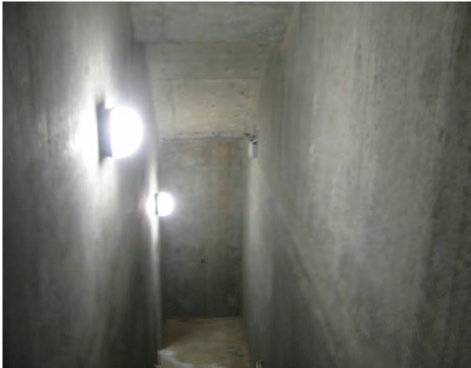
Photo 21 – LS11 – The south stairwell at the Ozonation Basin has no dedicated ventilation.
