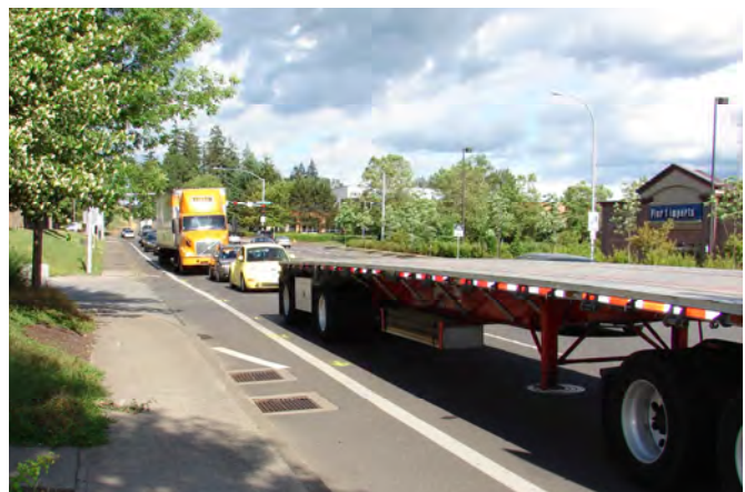
Roadway congestion and queuing on Elligsen Road leads to increased delay to freight movement.
