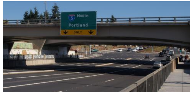
Looking east to the I-5/Wilsonville Road interchange.
