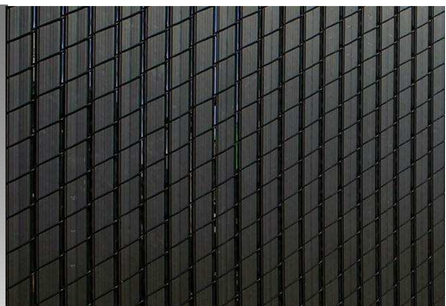
EXISTING AND PROPOSED FENCE TYPE: BLACK PAINTED CHAIN LINK WITH DARK GREY PLASTIC SLATting
