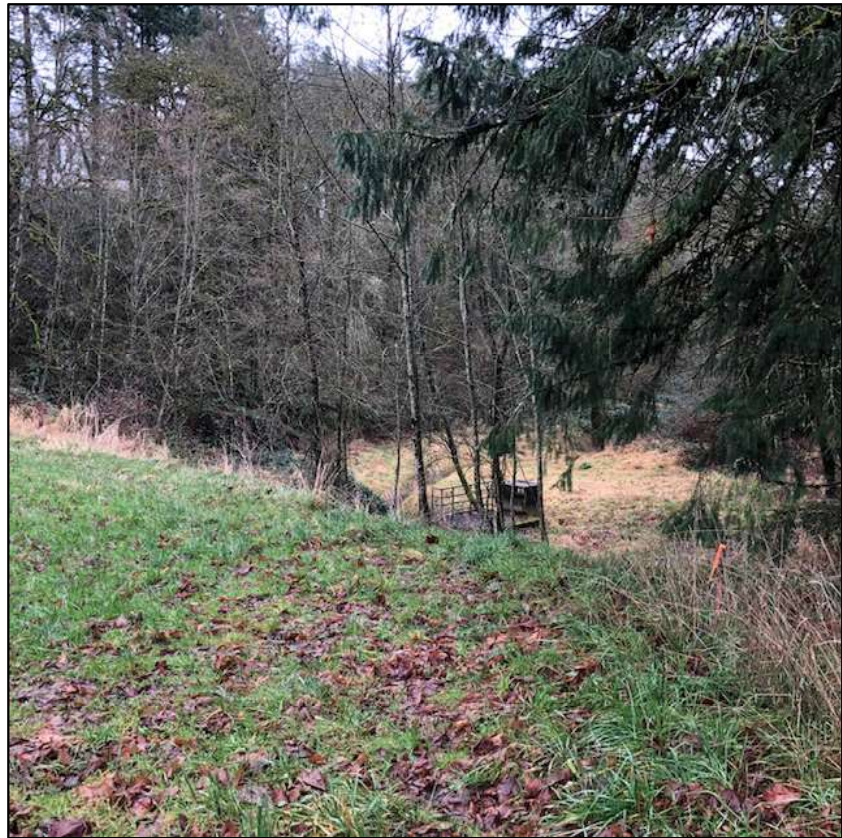
Upper Bench Looking Down at Creek and Flow Control Structure
