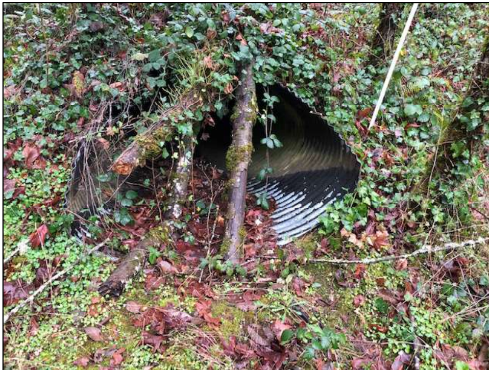
Emergency Overflow Culvert (42"x66" CMP - Corrugated Metal Pipe) Located on Upper Bench
