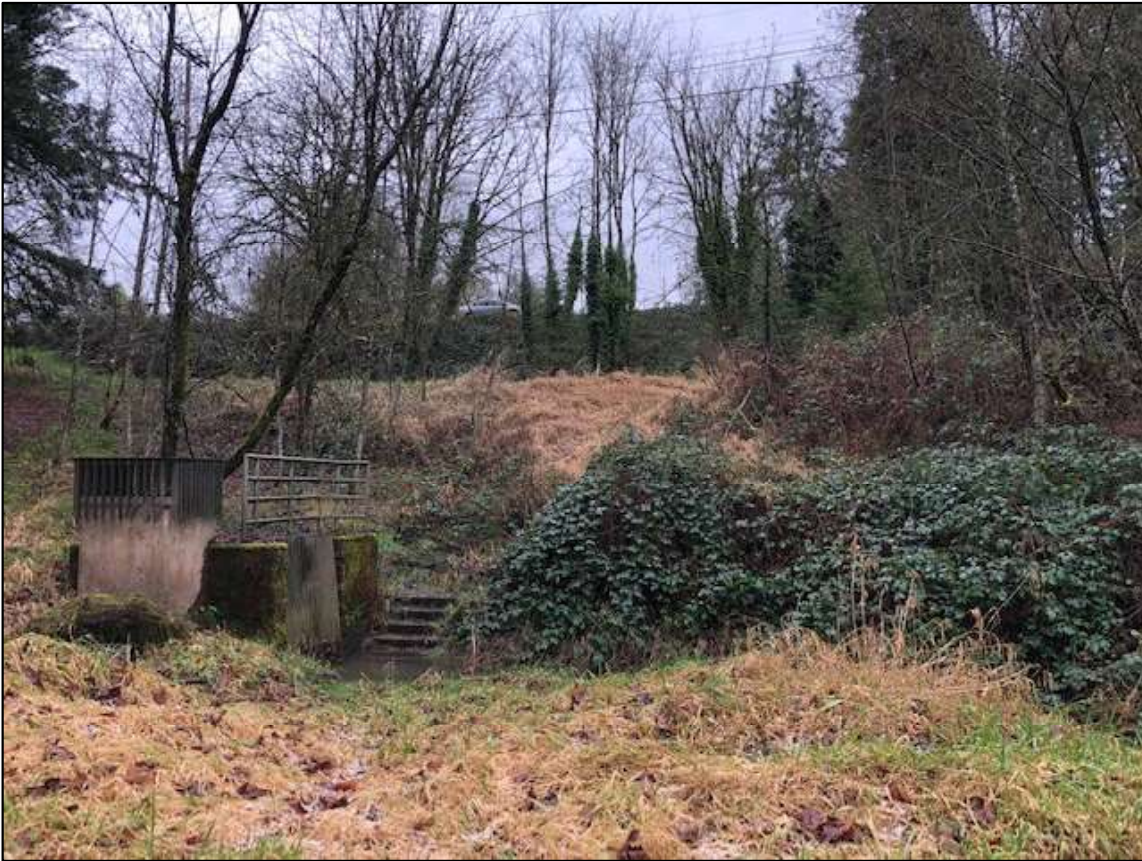
North to South View from Boeckman Creek up to Boeckman Road – Shows flow control structure for culvert and creek level, upper bench and road (see car)
