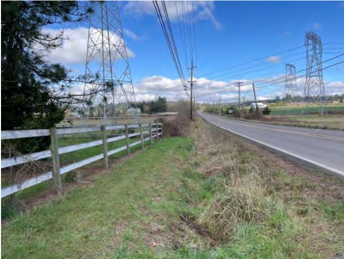
Photo A. View north of roadside ditch along Stafford Road.
