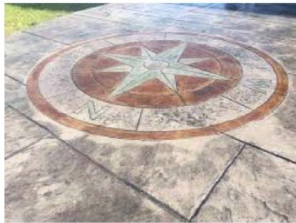
EXAMPLE OF STAMPED CONCRETE SCALE: NTS
