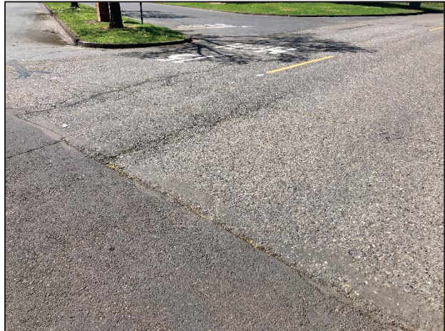
Photo 2: North Entrance Drive – Fatigue Cracking and Raveling. Note sealcoat on eastern section of roadway.
