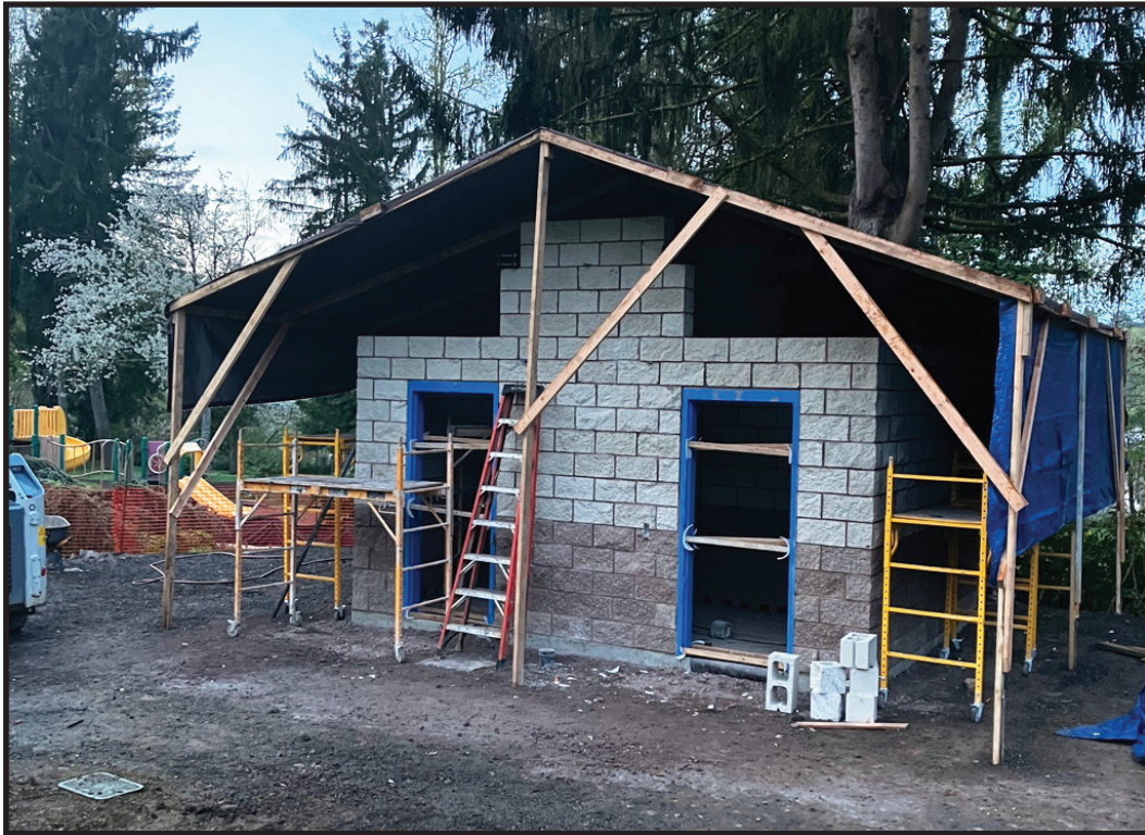
New restroom construction at Boones Ferry Park (CIP #9171).
