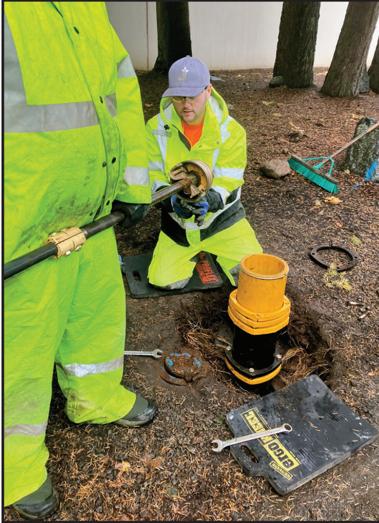
Water Distribution Technicians rebuilding a fire hydrant.
