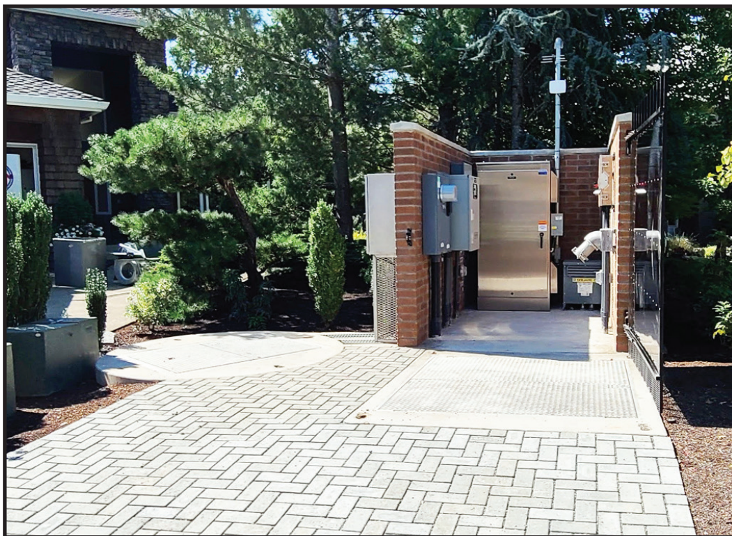
Final completion of the Corral Creek Sewer Lift Station rehabilitation (CIP #2105).
