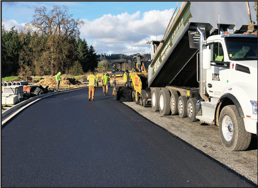
New roadway paving in Frog Pond West.
