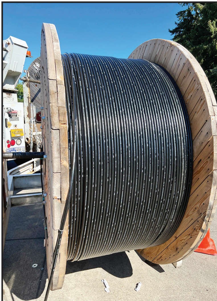
Spool of fiber for City infrastructure connectivity (CIP #8093).
