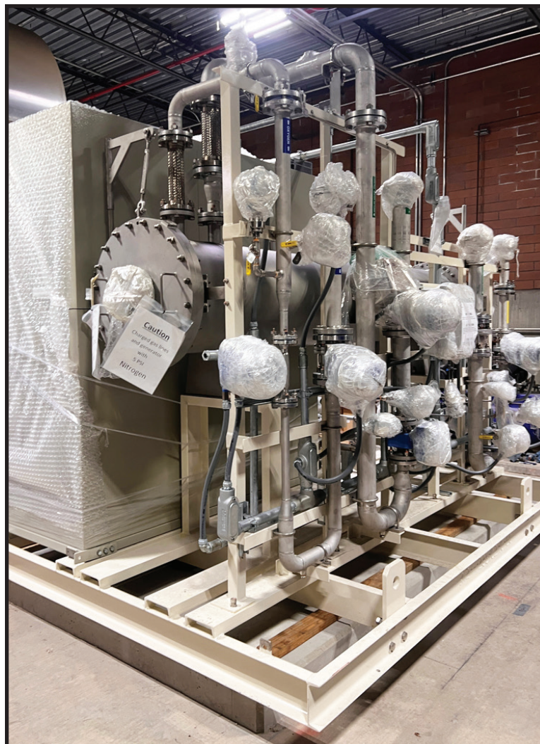
New ozone generator installation underway to expand capacity of the Willamette River Water Treatment Plant (CIP #1144).
