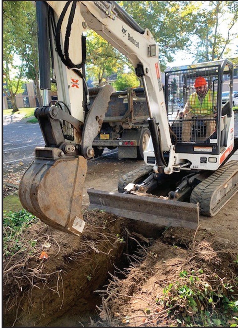
Stormwater staff performing storm main line pipe repair in Charbonneau.
