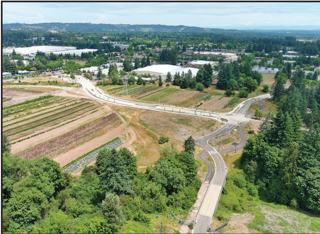
Aerial view looking northeast of a completed 5th Street/Kinsman Road Extension (CIP #4196).
