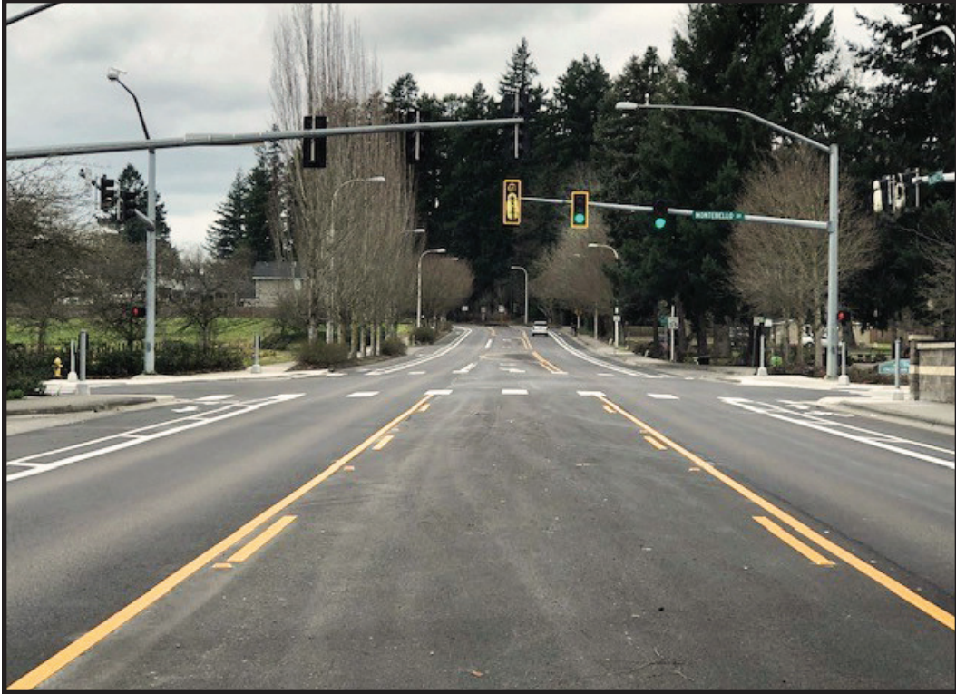
2019 Street Maintenance Program - Wilsonville Road
