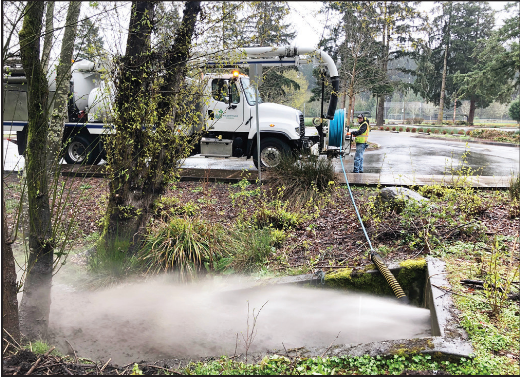
Cleaning plugged storm pipe
