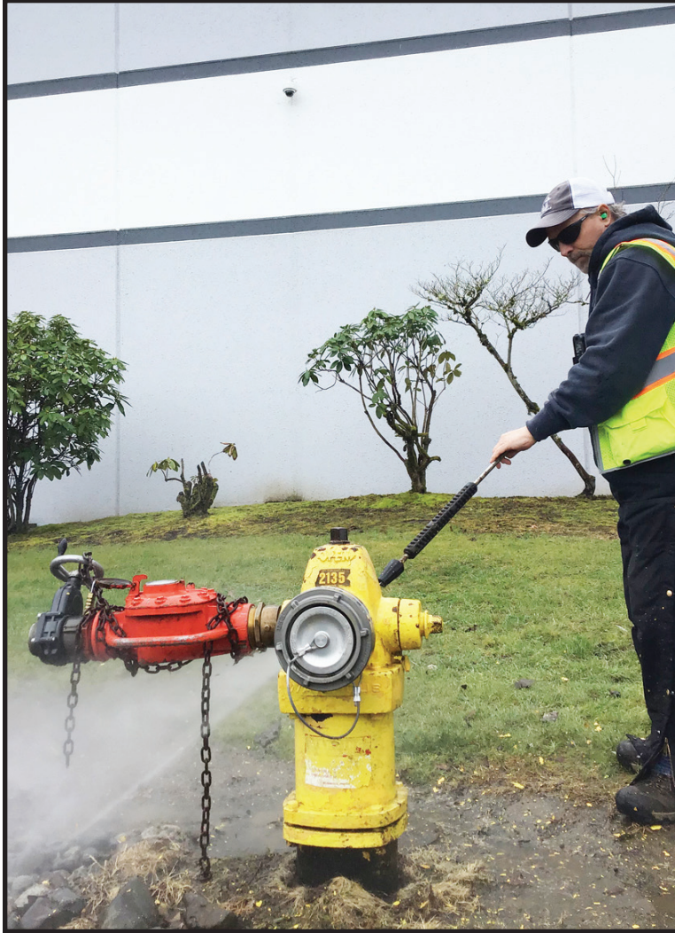
Fire hydrant cleaning
