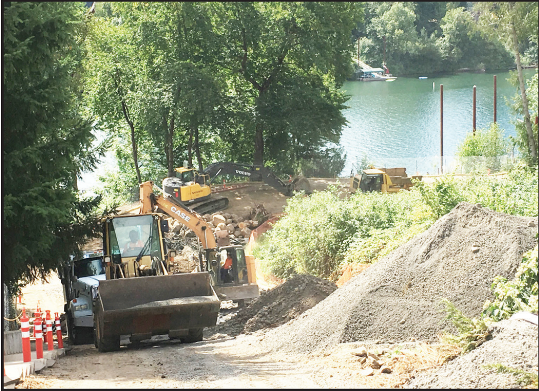
Belnap and Morey Court Outfall Restoration Project
