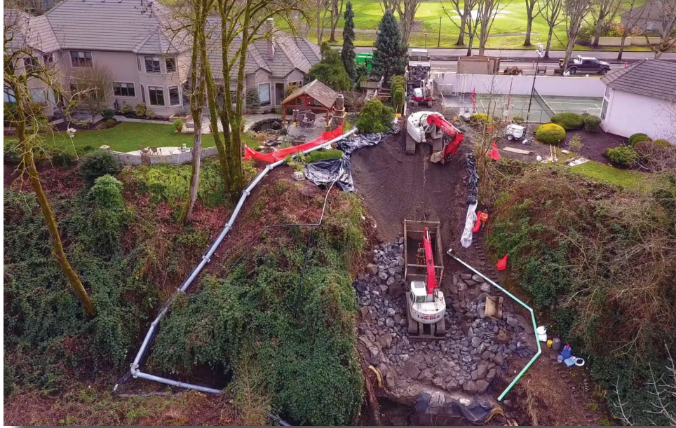
Emergency Outfall Repair
