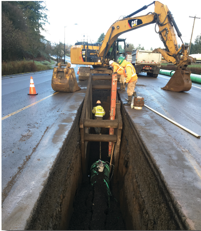
Tooze Road Improvements
