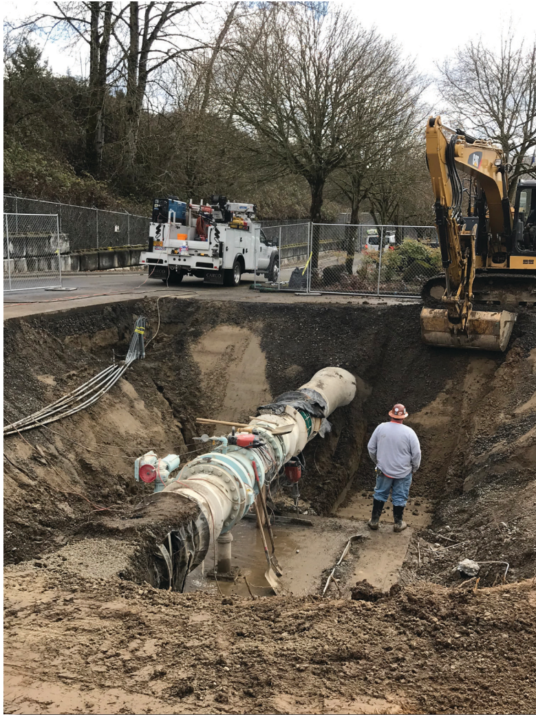
Vault Replacement at Water Treatment Plant
