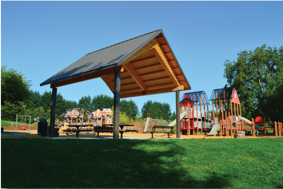
Murase Park Play Structure
