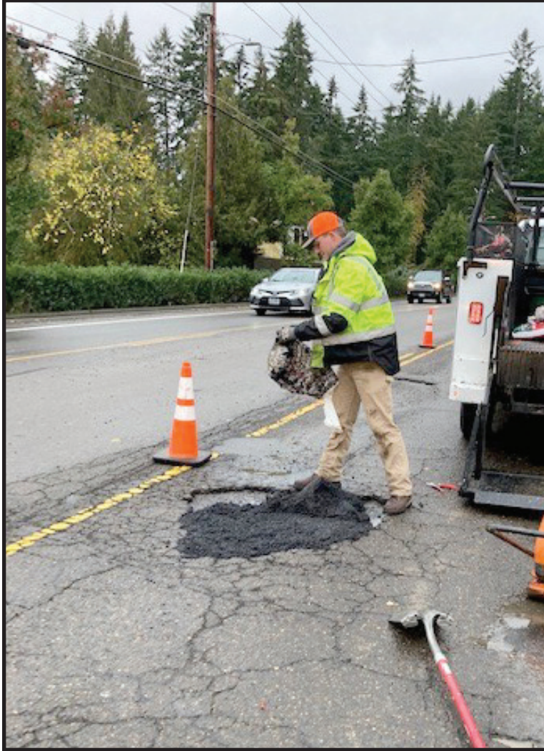
Roads staff using bagged cold asphalt patch to repair potholes.
