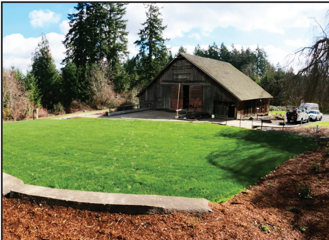
Improvement of the gathering space in front of the Stein-Boozier Barn at Murase Plaza as part of the Memorial Park Master Plan. Project was completed in-house for considerable savings (CIP #9132).
