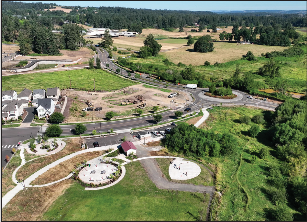
Regional Park 7 & 8 construction in Villebois.
