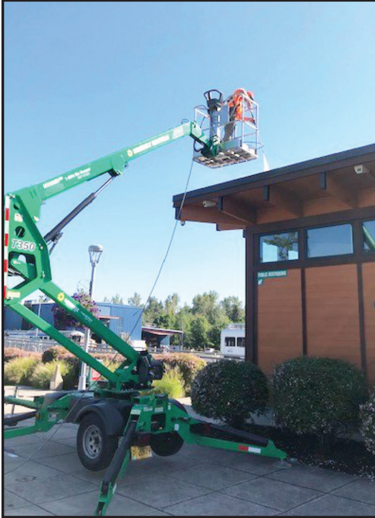
Facilities staff power washing a roof.
