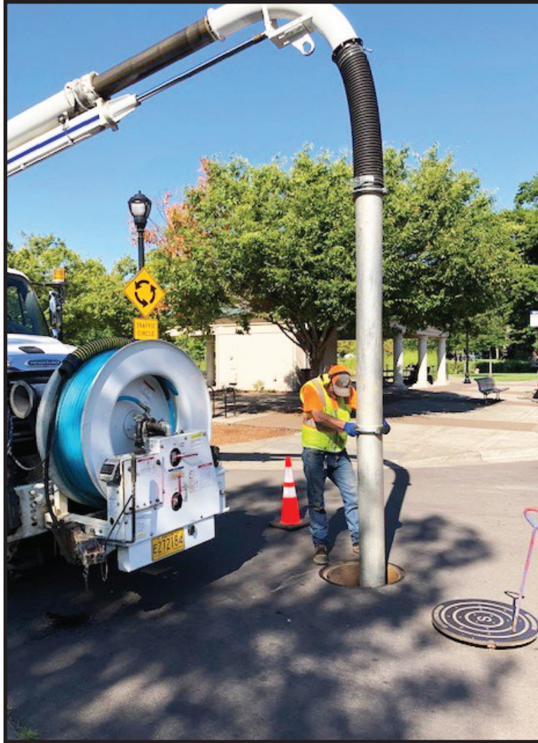
Stormwater staff cleaning a manhole.
