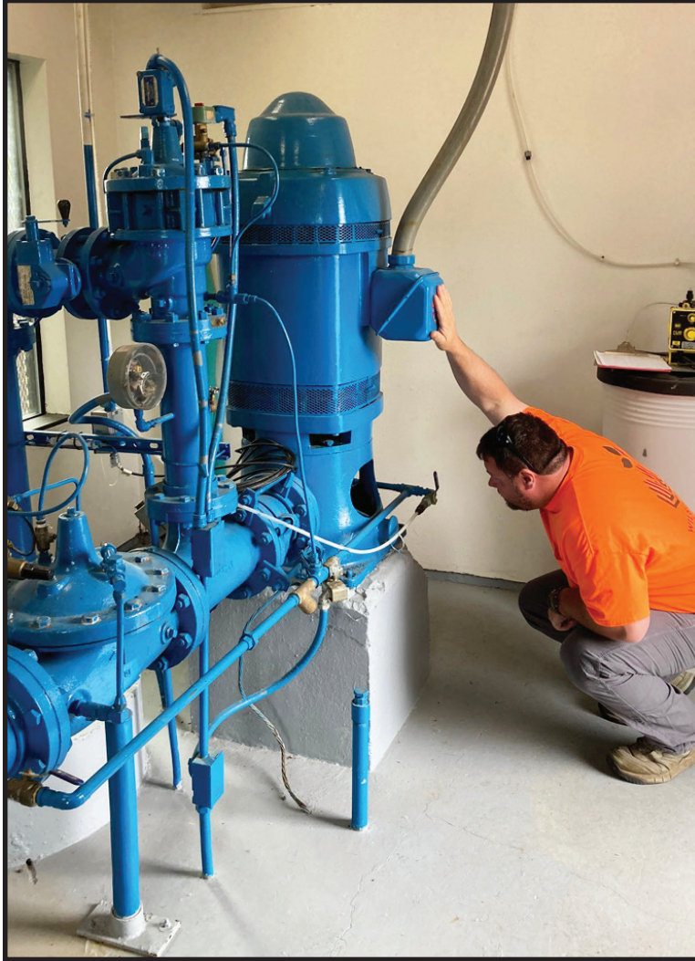
Staff inspecting the condition of water pump.
