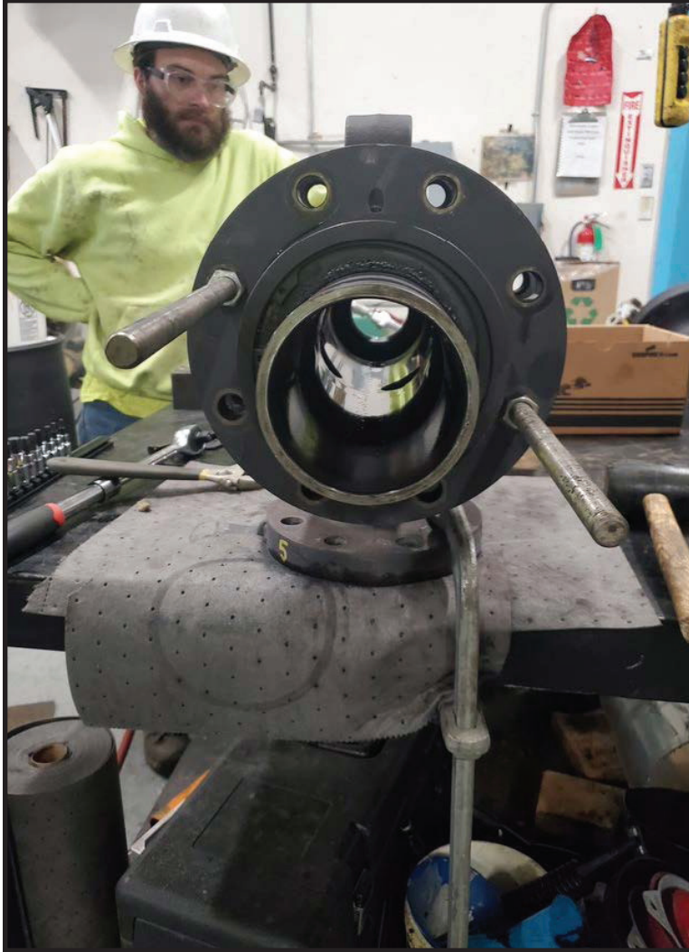
Jacobs staff rebuilding biosolid dryer valve.
