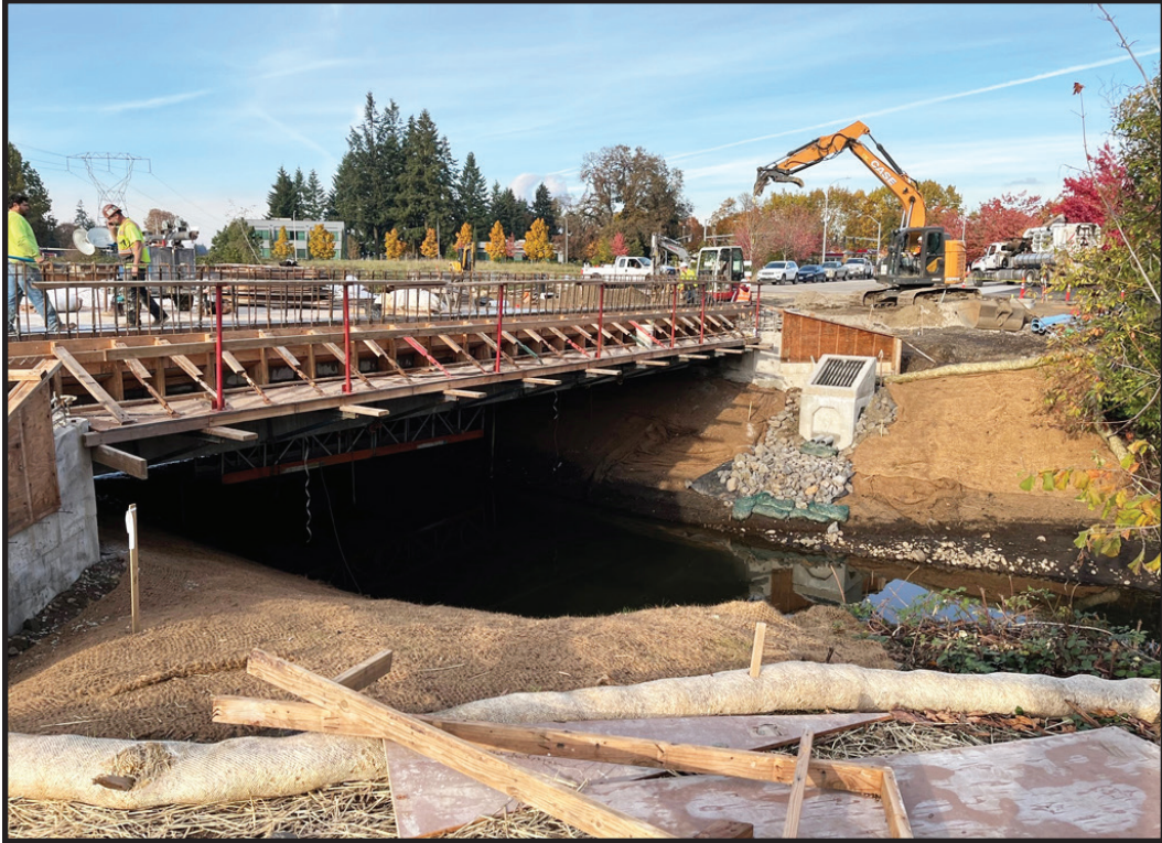
Kinsman Road bridge construction over Coffee Creek.
