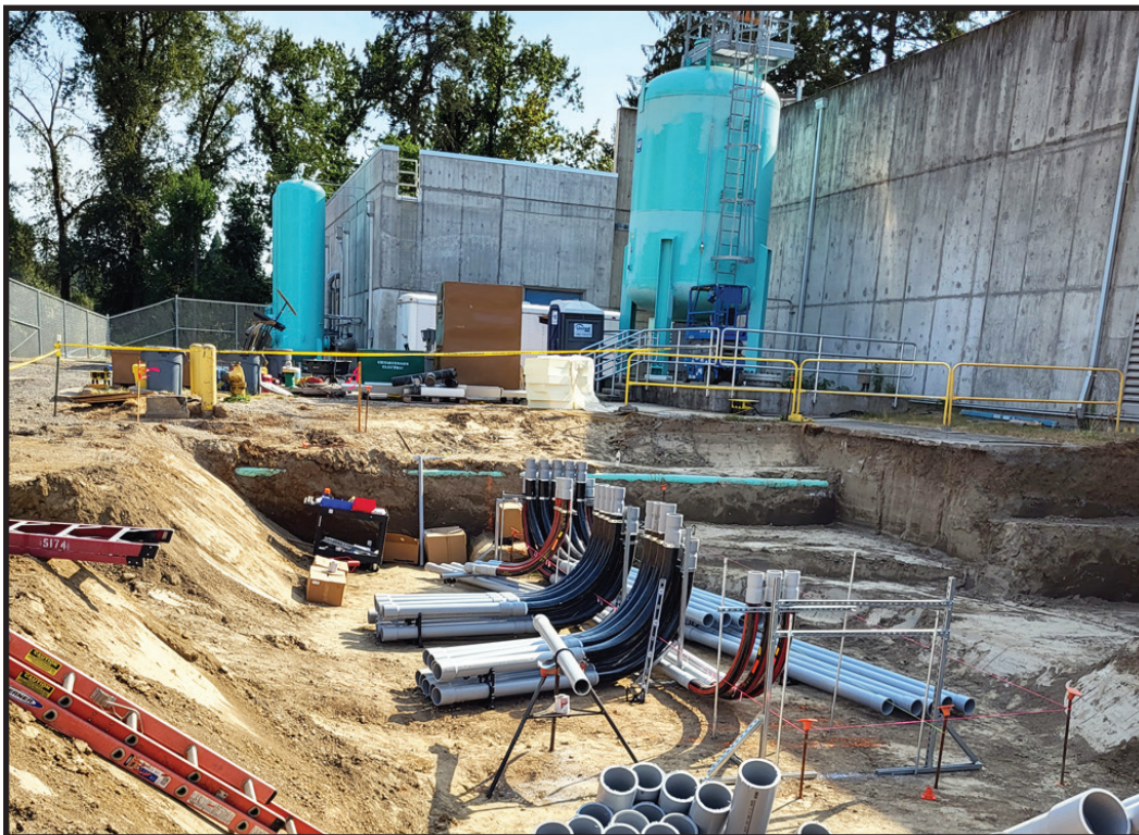
Conduit being installed for the Water Treatment Plant expansion (CIP #1144).
