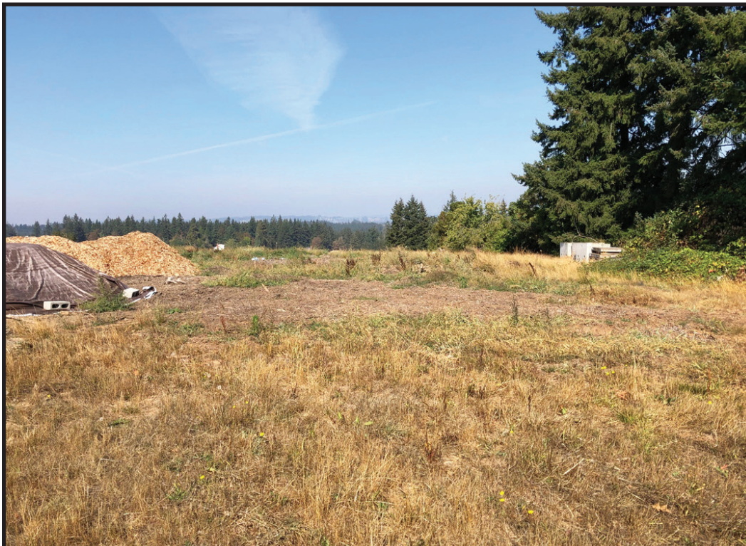
The existing site prior to construction of the West Side Level B Reservoir (CIP #1149).
