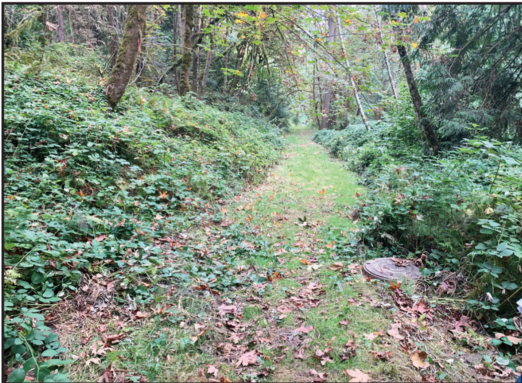
Existing sewer manhole and unimproved access path around Boeckman Creek (CIP #2017).
