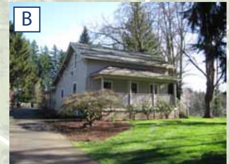
B The Tauchman House was the residence of ferry operator Emil Tauchman. The house later served as Wilsonville City Hall from 1971 to 1976. Available for rent through Community Center!
