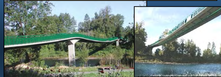
Grants Pass Ribbon Bridge
