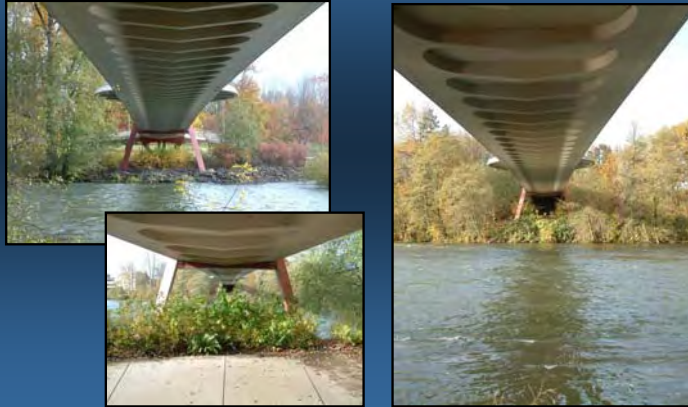
Walkway and under-deck of DeFazio Bridge
