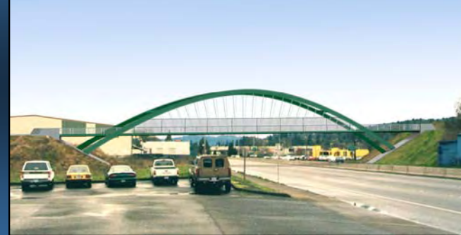
McLoughlin Pedestrian Bridge in Portland (under construction)
