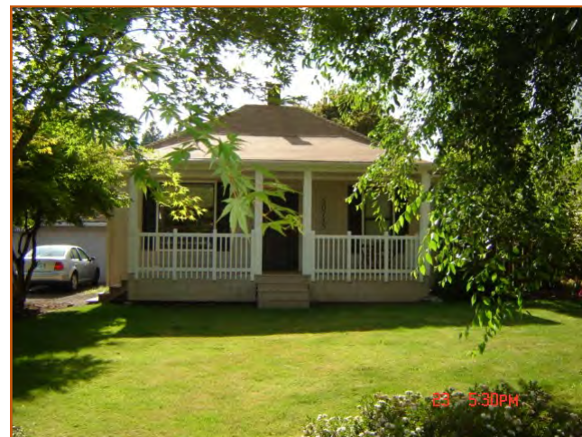
STATIONMASTER HOUSE 19?? (moved here)
