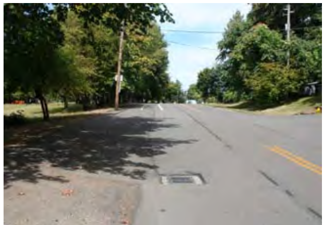
Existing Road Includes Curbless Street, Bike Lane and Remnant Orchard
