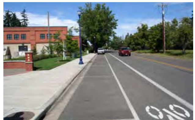
Existing Road Includes Sidewalk, Parking, and Single Bike Lane
