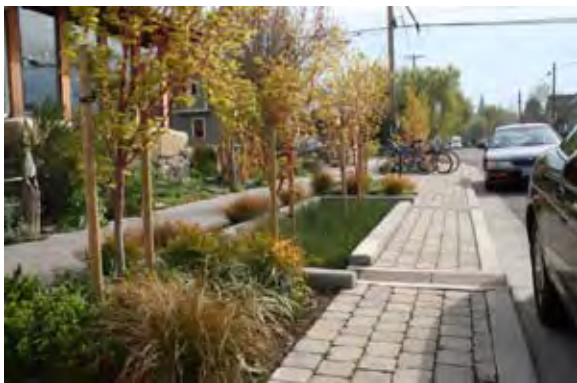
Stormwater Planters and Street-Side Parking Example
