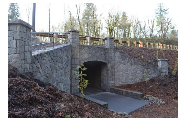
UNDERCROSSING EXAMPLE 2: SR-14 Tunnel in Skamania County, WA
