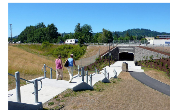
After: South end of SR 14 Pedestrian Tunnel, with stairs and ADA-accessible path connecting to fitness trail along the top of the Columbia River dike
