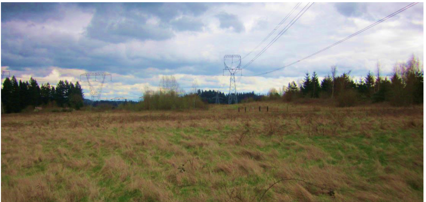
Figure 28. Existing BPA Corridor
