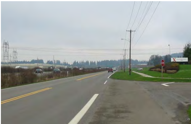
Parkway Avenue near the Xerox campus is a Minor Arterial but does not include bike lanes. There is a sidewalk on the east side, but it ends at the boundary with the vacant parcel to the north.
