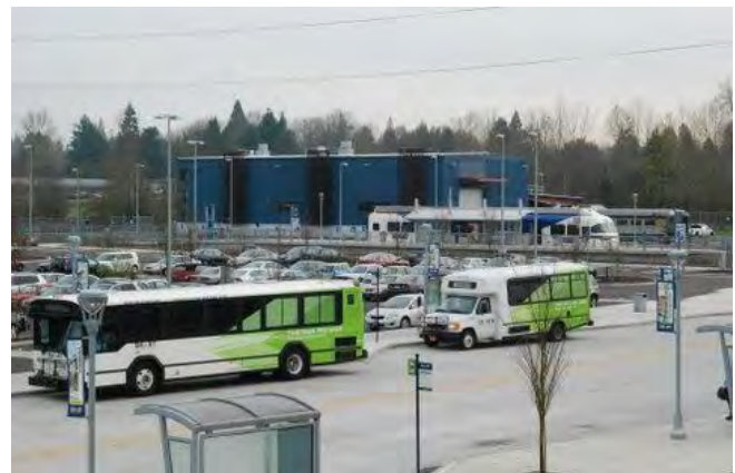
Wilsonville's transit center, SMART Central at Wilsonville Station, is located at the corner of Baber Street and Kinsman Road. It is SMART's main transportation hub and includes a 400-stall park-and-ride lot, twelve bus bays, an operator break room, public restrooms, shelters, and a clock tower with security cameras. It also shares the site with TriMet's Westside Express Service (WES) commuter rail station. Wilsonville is WES's southern terminus.
