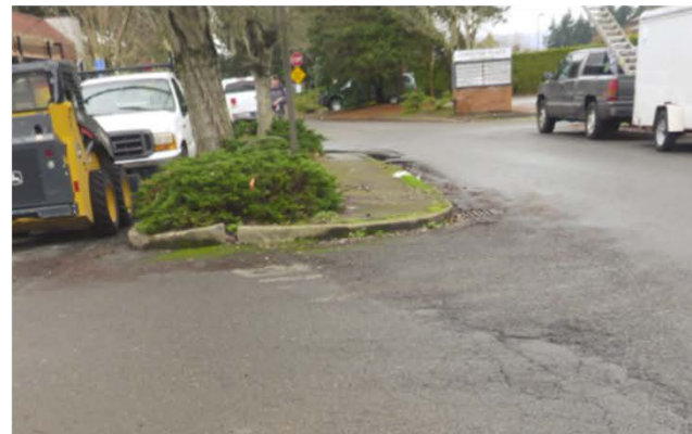
Crossing location at Driveways Top - LTS 1 at Wilsonville Medical Plaza Middle - LTS 2 at Northwest Rugs Bottom - LTS 3 at Starbucks onto Citizens Drive
