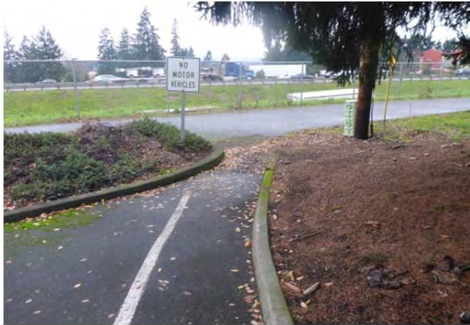
Looking west at the access from Citizen Drive to the multi-use path west of Town Center Loop
