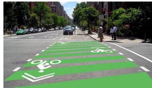
Cycle Track Crossing
