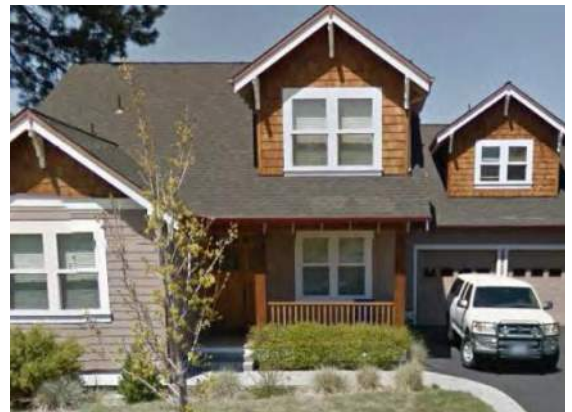
Recessed garages help to create a more attractive neighborhood street.
