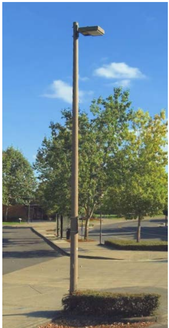
Shoe Box Light Pole Acceptable:
