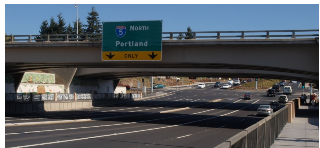
Looking east to the I-5/Wilsonville Road interchange.
