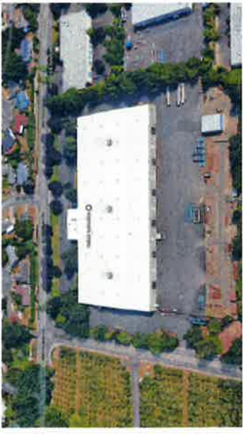
BUILDING DESIGNATION D
