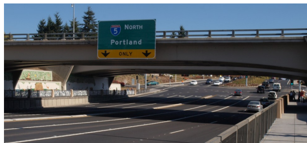
Looking east to the I-5/Wilsonville Road interchange.
